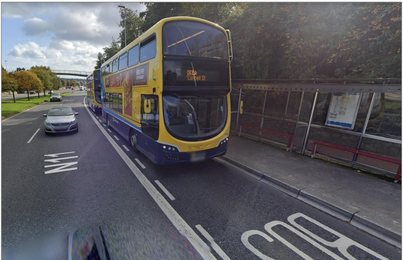
Figure 7.2 Where space permits double bus bay should be provided where more than one bus is expected to arrive at a bus stop simultaneously (source: Google)
